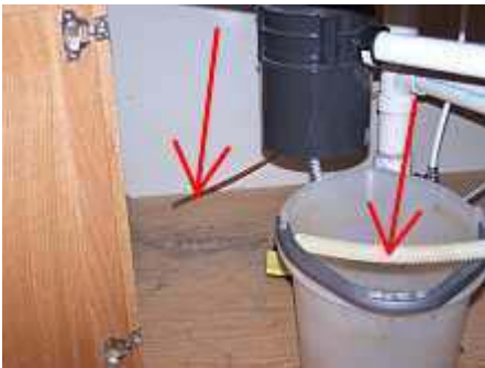
Photo 32 Dishwasher line not attached
